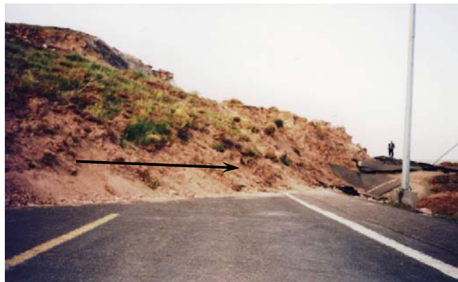
Figure 3. Road displacement accompany the moved mass
