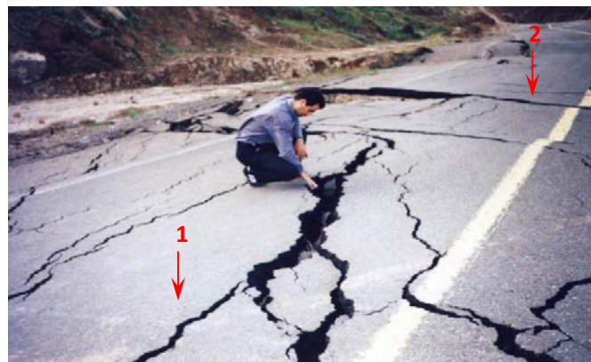
Figure 5. Tension fractures (!) and shearing fractures (2)
