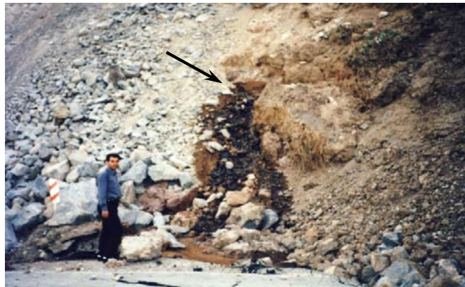
Figure 6. A new spring formed in the movement location
